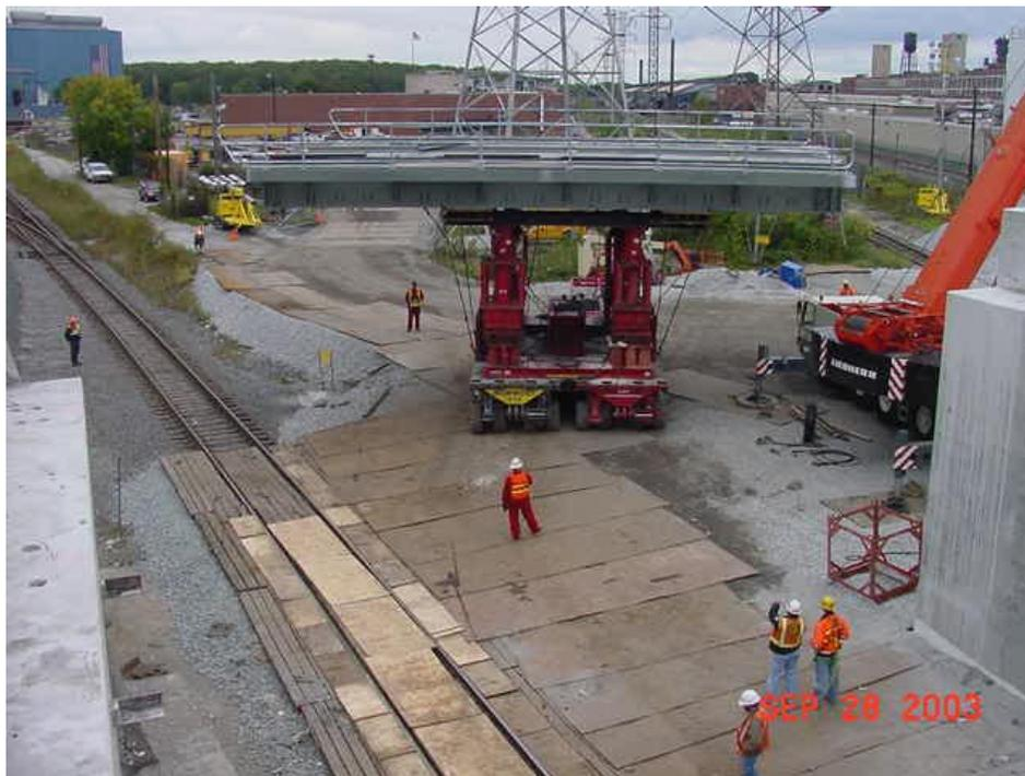
So you want to move a bridge! On September 28 Kiewit Western hired Mammoet Systems to move in the two bridge structures at the Metra bridge crossing over CSX and NS at Riverdale. Shutdown started at 7 PM on the 27th, at 2 PM the contractor started moving the bridge from the parking lot and set in place over CSX, ready for track, around 5 PM on the 28th. NS was finished at 2 AM the following morning. Photo by R. Schroeder
