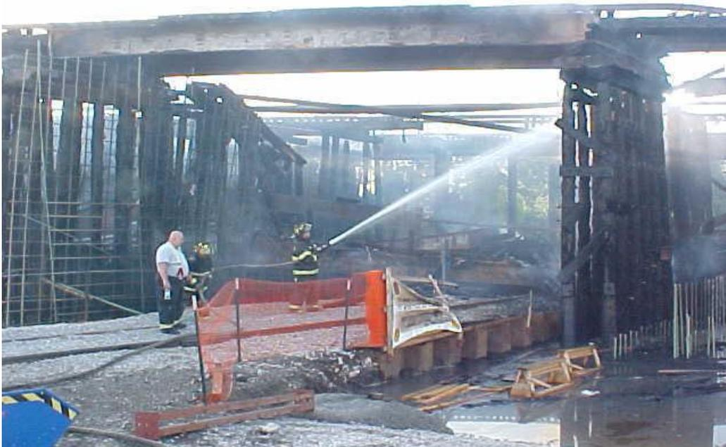
Sunday night, June 22, 2003, fire destroyed two timber trestles owned by Metra and four owned by the CNIC at Riverdale, Illinois. A contractor was in the process of rebuilding the two Metra bridges with roll in planned for Labor Day weekend. The track shown is Norfolk Southern, former PRR track, that serves a nearby steel mill. - Photo by CSX
